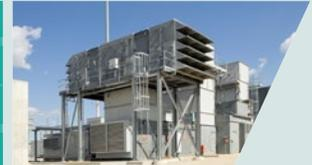
ECG 2.1.13 Natural Gas-Fired Reciprocating Engine System—Cogeneration Mode
