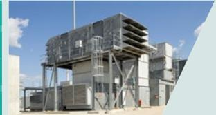
ECG 2.1.15 Landfill or Digester Gas-Fired Reciprocating Engine System—Cogeneration Mode
