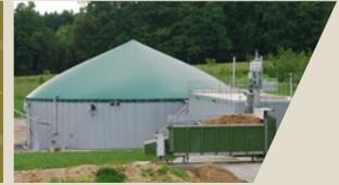
**BGS 2.14.1 System to Produce Biogas by Anaerobic Digestion of Organic Waste**
